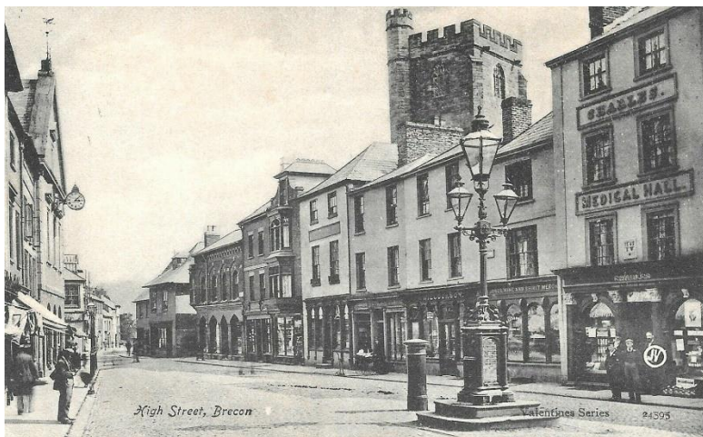
Gas Lamp. Brecon High Street
